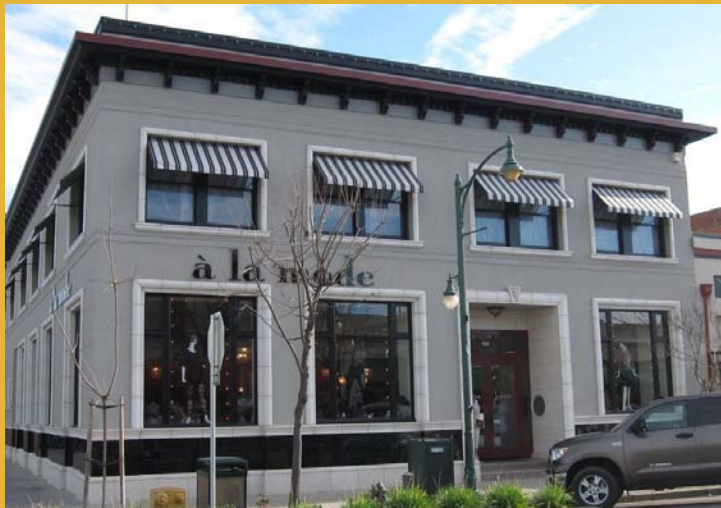
Bank of America Building after rehabilitation, 2010, Exeter, CA (courtesy of Johnson Architecture)
