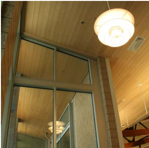
Port orford cedar runs fluidly from interior to exterior along the West reading area.
